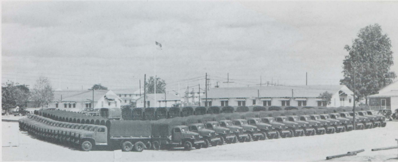
PART OF MOTORIZED EQUIPMENT
