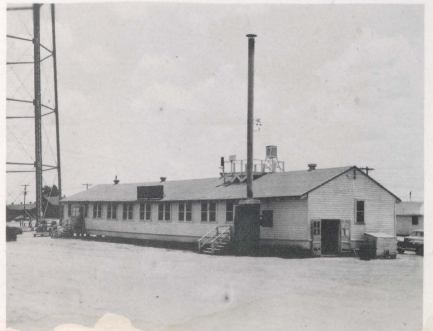
MESS HALL AND KITCHEN BUILDING
